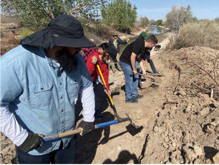
Image 11. Students work alongside volunteers to level out a water channel to allow for more water flow and bank inundation once water is released into the wetlands. Photo Credit: Dr. Ramos-Chavez
